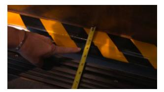
Measure and write down the distances between the landing door and the running clearance on each of the left side and the right side of the landing door.
